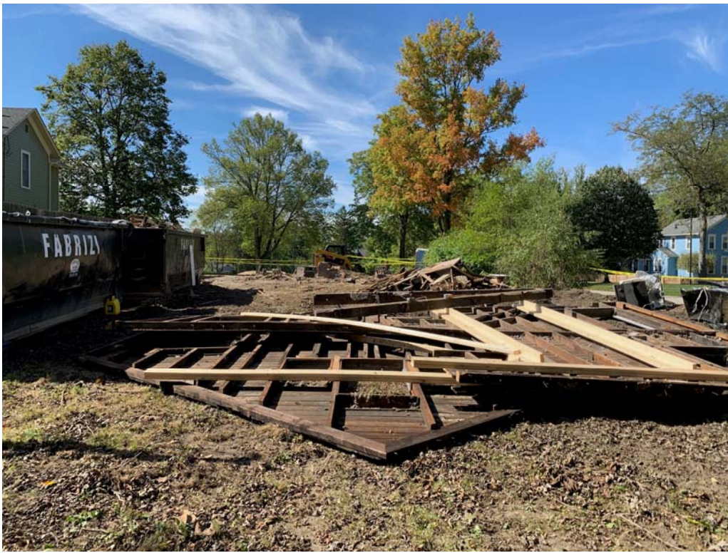
Demolition of the 37 North Oviatt Street House on October 4, 2019.
